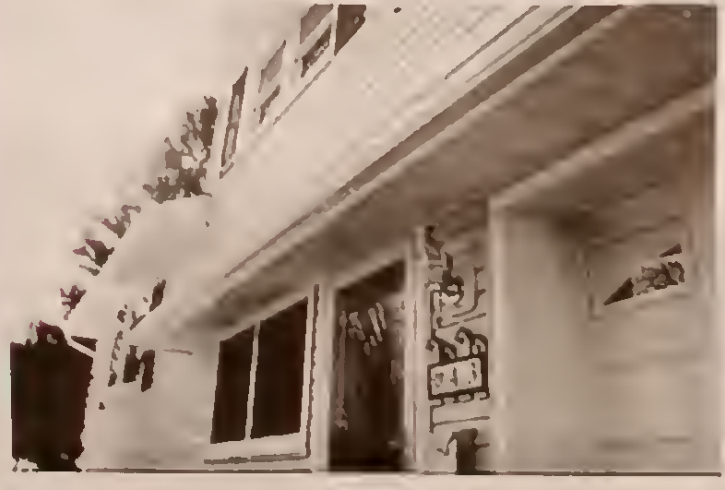
VINYL SIDING REPLACEMENT WINDOWS
