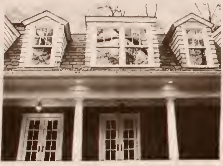
WOOD SHAKES MANOR ROOF
