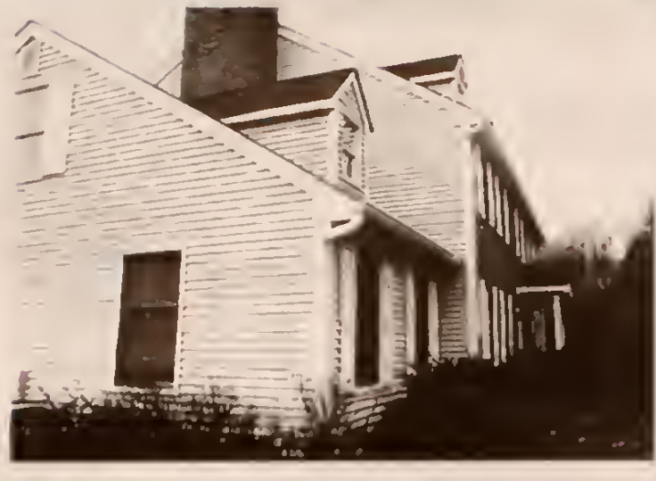
VINYL SIDING ASPHALT ROOF
