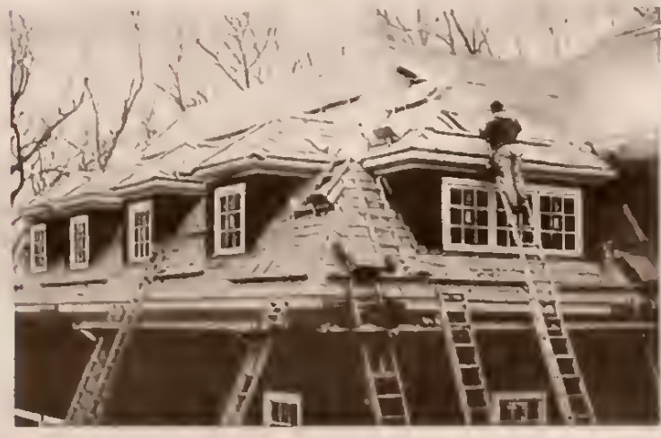
SLATE ROOF COPPER WORK
