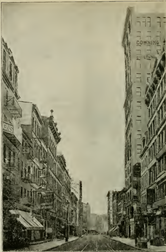
LOOKING DOWN FULTON STREET.
