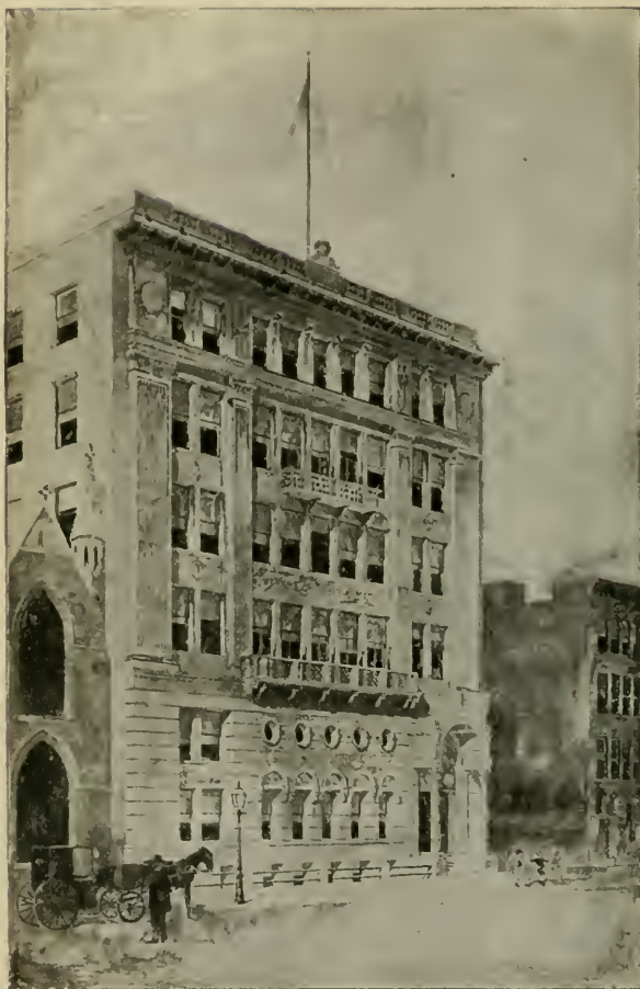
NEW BUILDING OF THE COLLEGE OF PHARMACY.
