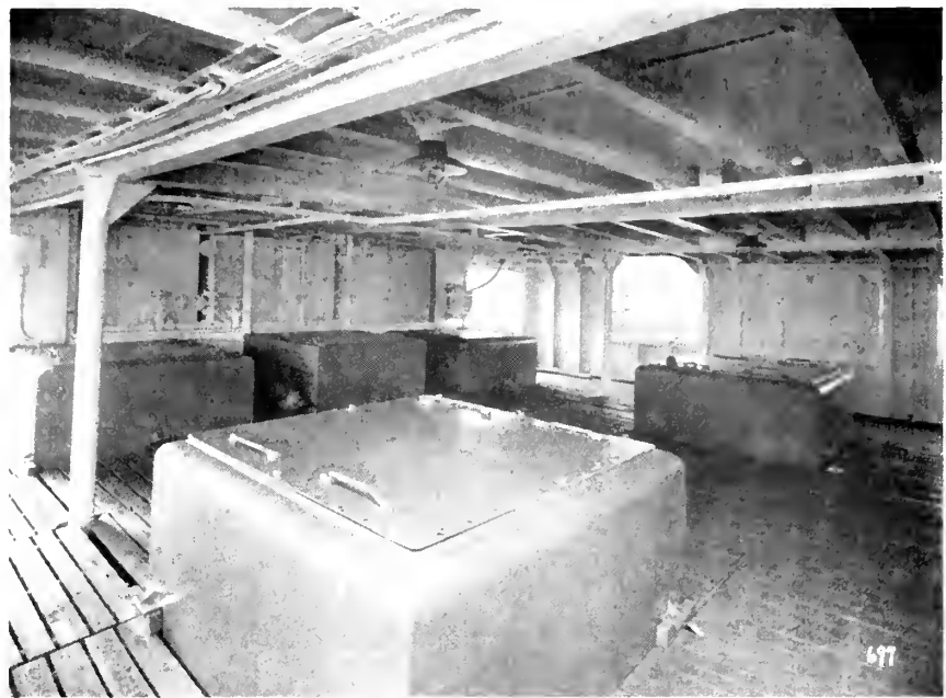
Steel hatches to fish and bait tonks on sheltered main deck.
