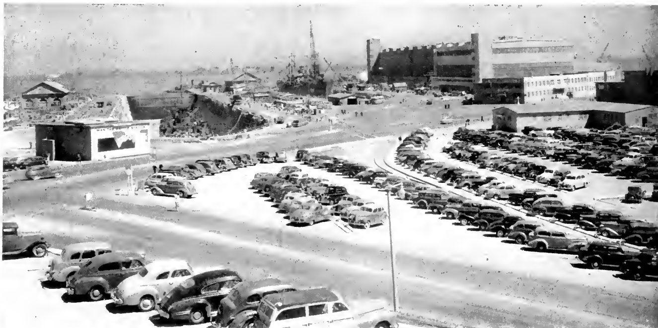
Fig. 1: The two original docks, huge machine shop and parking lot.
