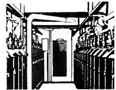
CARBON DIOXIDE CYLINDERS
