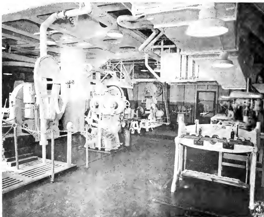
Sheet Metal Shop.
