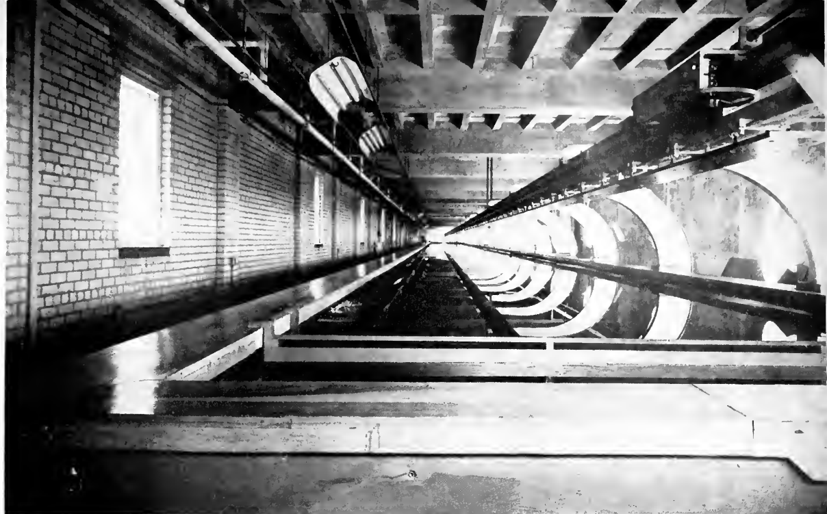
View of No. 3 tank room, showing rail supports and towing cable
