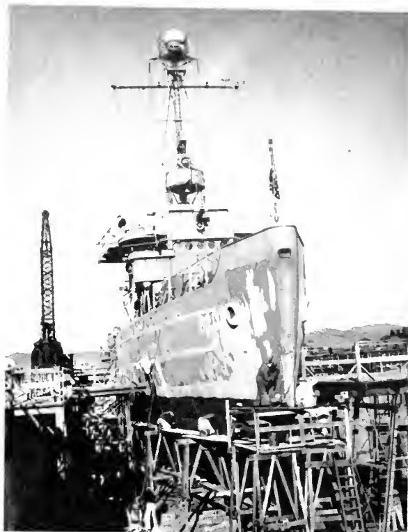
MINESWEEPER UNDER REPAIR IN ONE OF YARD'S DRYDOCKS
