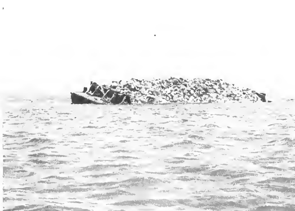
Below, left: A cargo of stone being unloaded from side-dump tilting barge. The barge is self-dumping and requires about 17 feet of water in which to operate, and bails itself at the end of each operation. Below, right: A big clamshell dredge at work dredging inner harbor.
