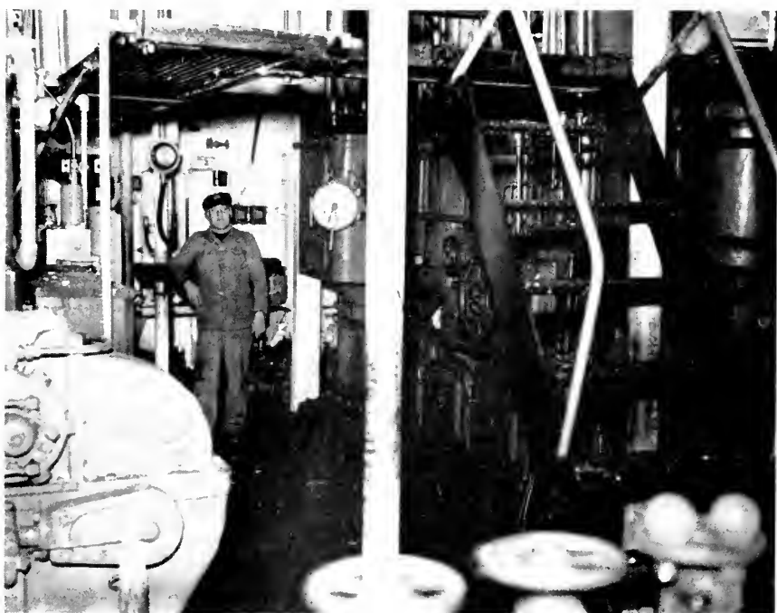
The Foz Do Douro's engine room.
