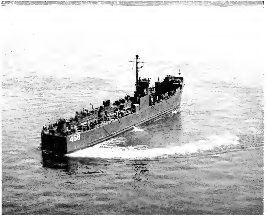
Upper: Equipped with the revolutionary new cycloidal propeller, view of the Navy LSM 458 in the process of executing a 360-degree turn without forward motion during recent tests in Puget Sound near Bremerton. The propeller also makes it possible for ships to move sideways and to come to a crash stop in a few seconds.
