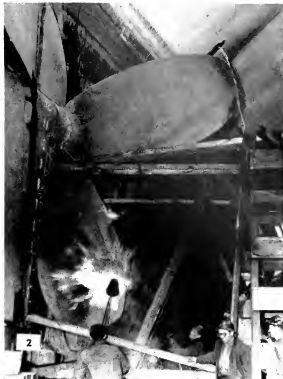
(1) Army transport George W. Goethals, converted to carry war brides, re-enters Todd Brooklyn division for repair of damaged propeller as shown in (2) where the torches heat the damaged propeller. A quick repair job sent the Goethals back to Europe on April 29.
