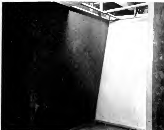
Fig. 1. Aetna all-steel bulkheading and linings in place.
