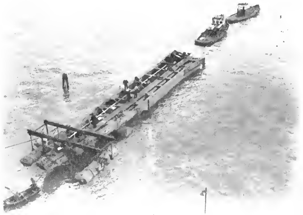
125' long digging ladder for dredge Papoose shown after being launched at Bethlehem's San Francisco Yard. The ladder, which had been lengthened from 90' to 125', was then installed in the dredge.
