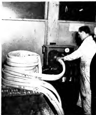
Coupling fire hose with expansion ring coupling.
