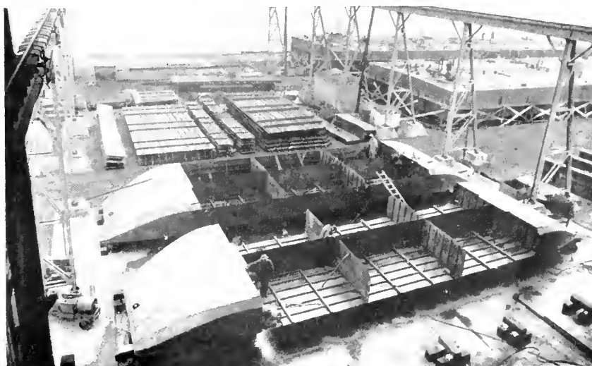
Oil barges under construction at Decatur Plant of Ingalls Shipbuilding Corp.
