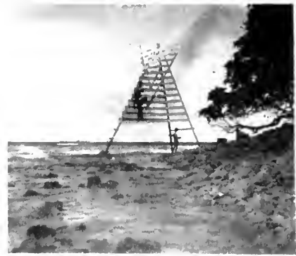
Strong, well-placed wire guys are the best insurance against the tripod tipping over in a typhoon.
