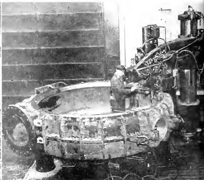
Below, right: Drilling and tapping 1 \frac{1}{2} " diameter stud holes for cover plate in 30" dredge pump casing for suction dredge San Diego. Work being done on drill press in machine shop at Bethlehem Steel Company's San Francisco Yard is typical of unusual jobs performed at this yard. Casing has a diameter of 9 feet and weighs approximately 14 tons.
