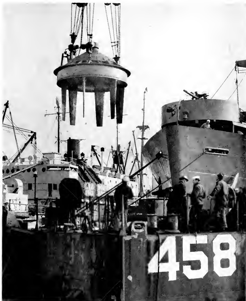
In the yards of the Everett Pacific Shipbuilding and Dry Dock Company one of the cycloidal propellers is being lowered into position on the Navy's LSM-458. Each propeller has an orbit diameter of 7 feet, and is equipped with six vertical blades, each of which revolves on its own axis as the rotor revolves.
