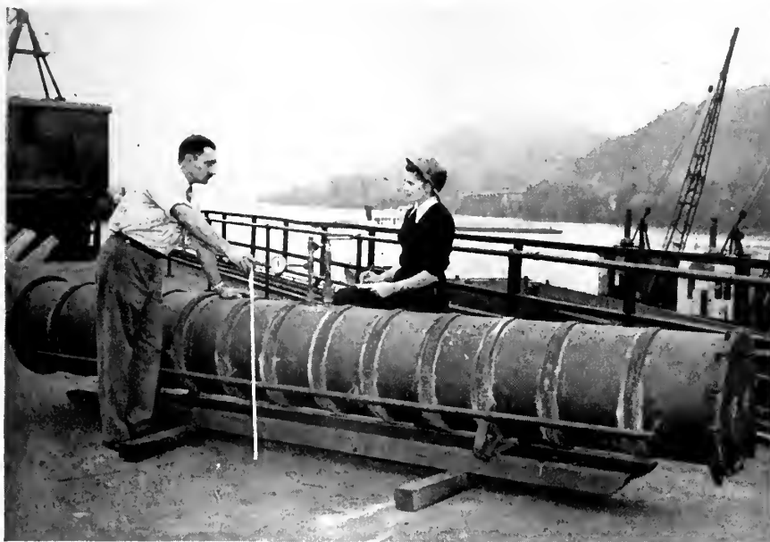
This 16-foot storage cylinder will house a height finder.
