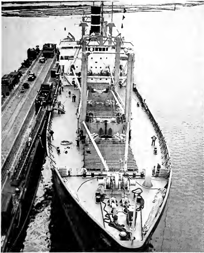
Shelter deck, forward, showing effected deletion of all armament. Wheelhouse top has also been cleared of that equipment. Minor changes were made in setting of cargo winches to improve operation of rigging.
