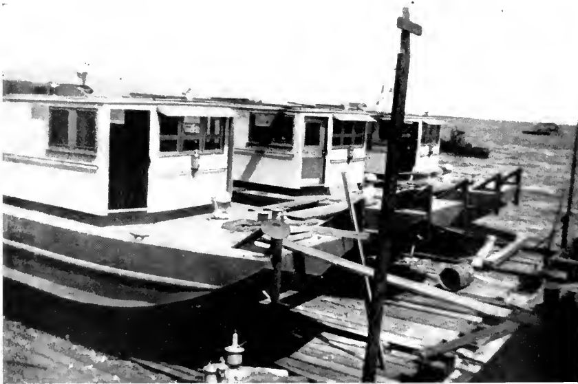
Above and right center: Four of the 16 house barges on the erection ways at Guira, eastern Venezuela.
