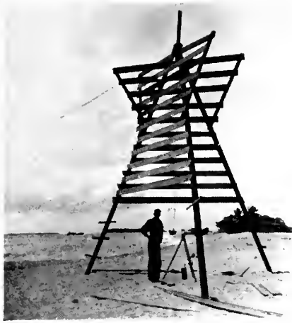
This beacon at one end of base line is placed on a sandy spit. In order to secure wire guys in sand, "dead men" are buried about three or four feet deep where necessary.
