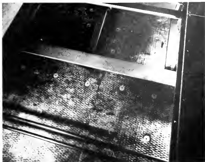
Fig. 4. View of overhead, Fiberglass insulation secured by Nelson nails.
