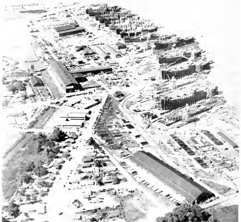
AERIAL VIEW OF INGALLS YARD —The sprawling Ingalls shipyard at Pascagoula, Miss., was busy on ships in all stages of construction when this aerial view was taken.
