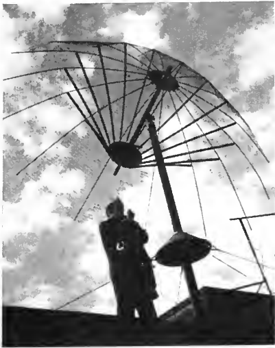
Typical of American radar equipment which smashed both German and Japanese armed might in the conflict begun just four years ago is this lightweight, portable unit developed by the Westinghouse Electric Corporation for the U. S. Marine Corps. Silhouetted against the sky is the unit's rotating "beach umbrella" antenna used as a reflector in sending out shortwave radio pulses and as a receiver to "catch" wave echoes reflected by enemy targets. Designed for beachhead use, the complete unit weighs only 400 pounds, can be dismantled and packed in four 100-pound cases, and has a range of 80 miles.
