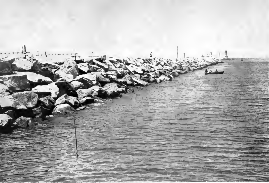
A long completed stretch of breakwater, showing level construction.
