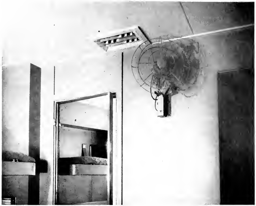
Fig. 3. View of type "R" special Agitair diffuser in small tourist class stateroom. (Courtesy Aetna Marine Corp.)
