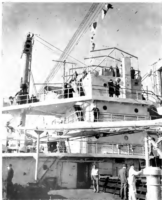
Looking forward at bridge superstructure. Port side.
