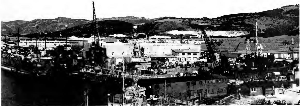
Section of the seawall. The four drydocks are on the far right.
