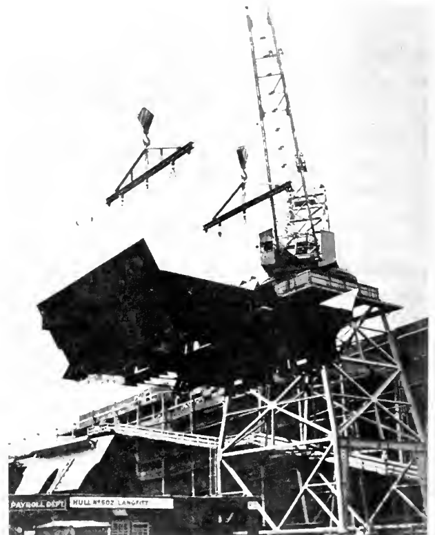
Two Gantrys swing a 55-ton hopper section aboard the Langfitt, huge all-welded dredge being built at the Ingalls Shipbuilding Corporation yards in Pascagoula, Miss., for the Corps of Engineers, U. S. Army. The sea-going dredge, one of four being constructed there at a cost of $4,250,000 each, will be 352 feet long—largest all-welded craft of this type ever built. The four dredges make up one contract among those for approximately $100,000,000 worth of construction on which Ingalls is now working.
