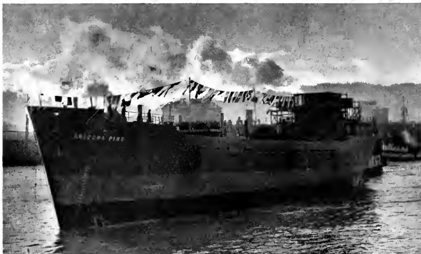
S. S. Arizona Pine, which was recently launched at Albina Engine & Machine Works. This ship is one of a series of lumber ships being constructed by Albina, featured in August 1945 Pacific Marine Review.
