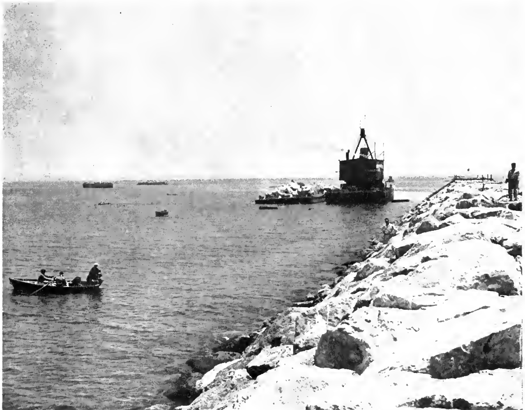
Derrick barge emplacing Class "A" stone on breakwater.
