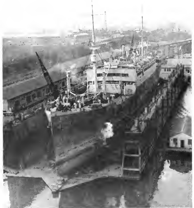
OFF THE BOTTOM of New York Harbor and safely dry-docked after narrow escapes in two World Wars, the Brazilian ship SS Pocomé is being repaired in U. S. Steel's Kearny, N. J. yard, to carry peacetime passengers and cargoes. Her stack and boilers had been removed for renovation before the photo was taken.
