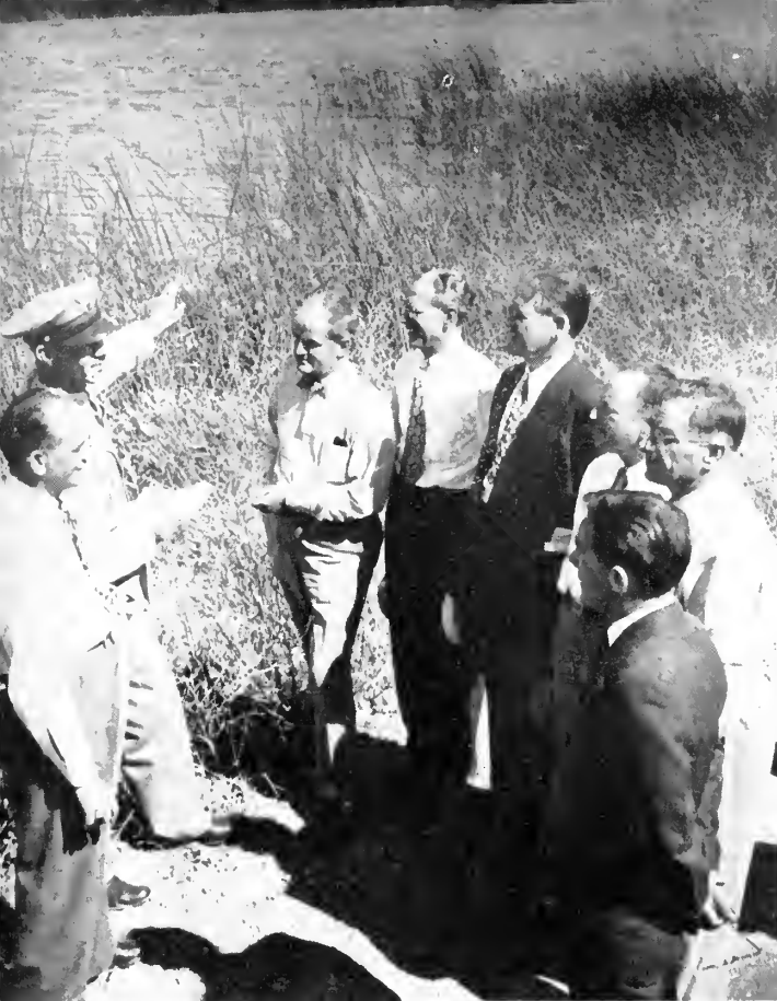
A group representing the House Committee on Rivers and Harbors making a physical inspection of the proposed ship channel course in the summer of 1945. Colonel Lester F. Rhodes, Sacramento District Engineer pointing out location of turning basin in Washington Lake.
