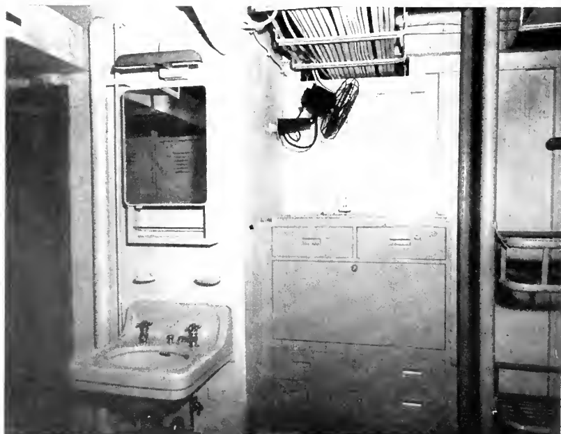
LOWER: A different arrangement of two berth cabin with bureau-desk lockers, and wash basin. Note joiner work on bulkhead.
