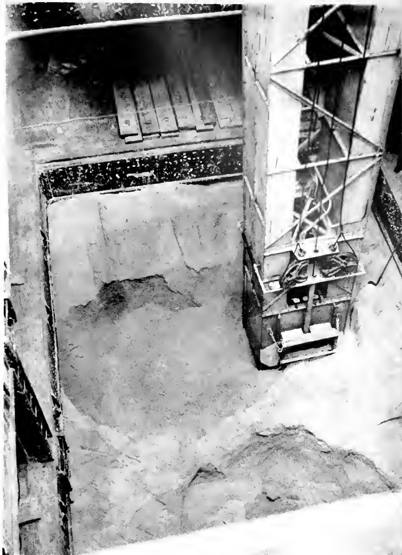
Bottom post of elevator which raises sugar from hold.
