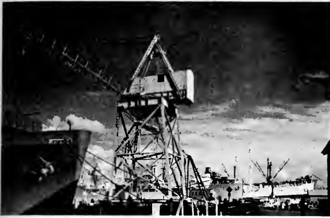
Waterfront facilities at Alameda yard
