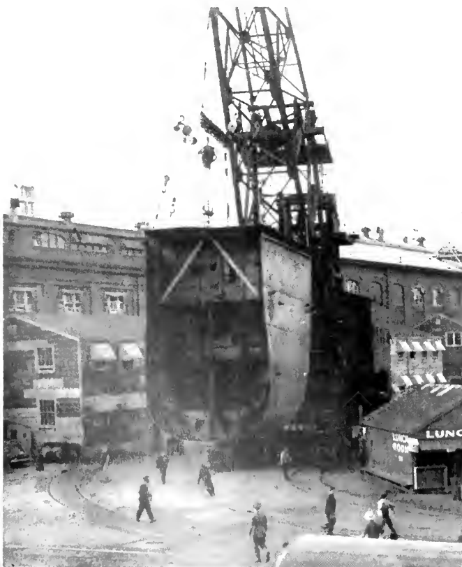
Slung from a traveling crane, one of the Pittsburgh's huge bow sections moves to the drydock. (Official U. S. Navy Photograph).
