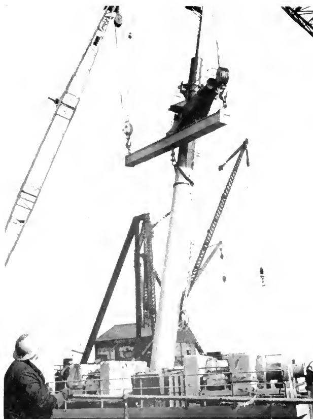
Stepping the mainmast on a 17,980 ton combined passenger and cargo ship for the American South African Line built at U.S. Steel's Federal shipyard at Kearny, N.J., is one of the heaviest lifts in the construction of pre-fabricated peacetime ships. Two cranes hoist the 42½ ton mast into place. It will be lowered through the tabernacle to the step upon which it rests below decks. (A tabernacle is a piece of large pipe braced with brackets to the lower deck.)
