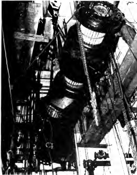
Fig. 4. Crankshaft being hoisted up through the ship's three decks.
