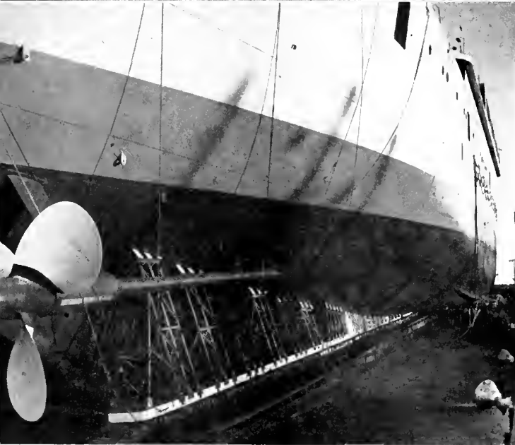
S.S. President Cleveland. View of hull from starboard after quarters with props removed ready for launching, showing propeller spectacle frame, and after poppet.
