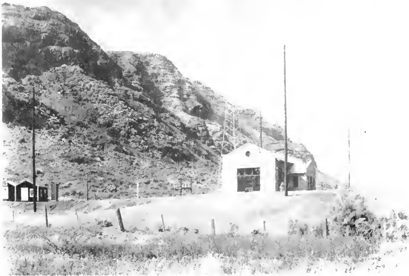
Koeno Point Transmitting Station, Globe Wireless Ltd., situated on northwest coast, Island of Oahu, 40 miles from Honolulu. From this station the first word of the tidal wave on April 1, 1946, was flashed to San Francisco.
