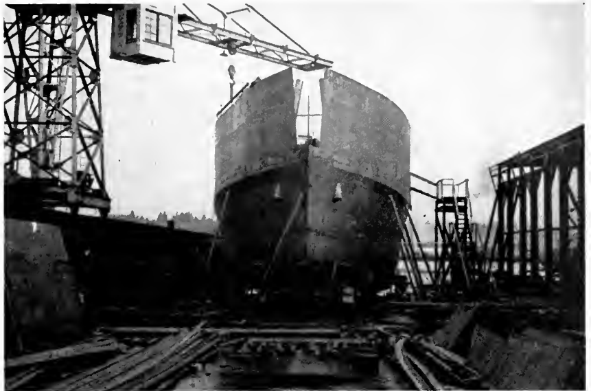
Setting shell around starboard bow above main deck.
