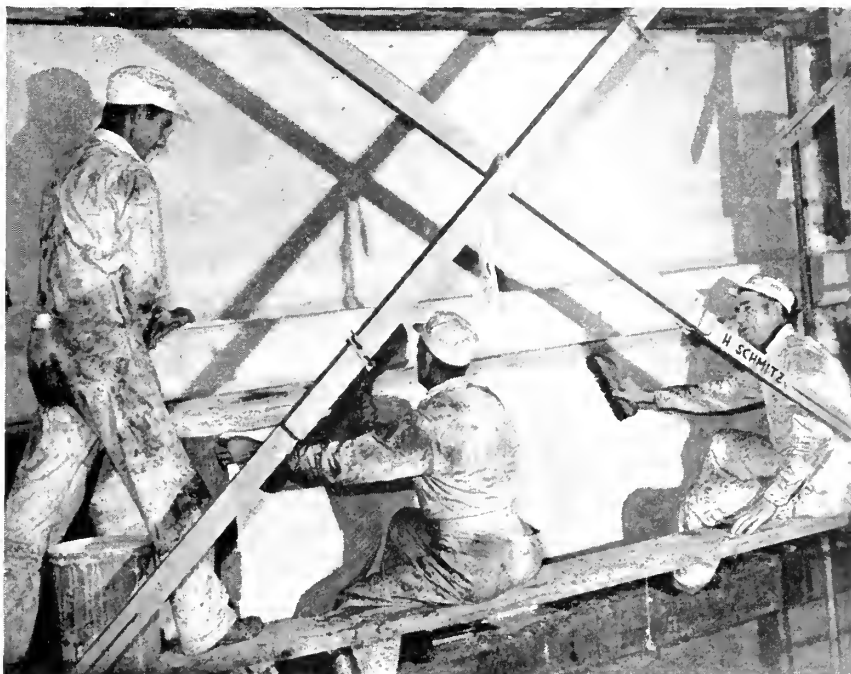
A lining installation.
