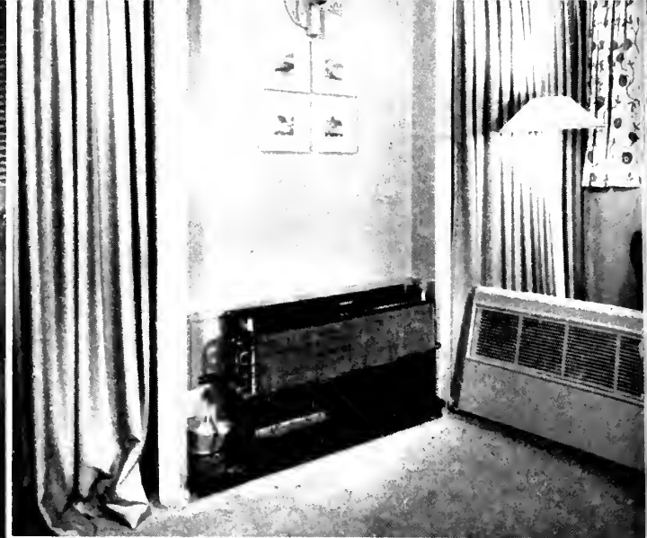
Fig. 6. View of Carrier air conditioning unit in large cabin class stateroom, enclosure removable.
