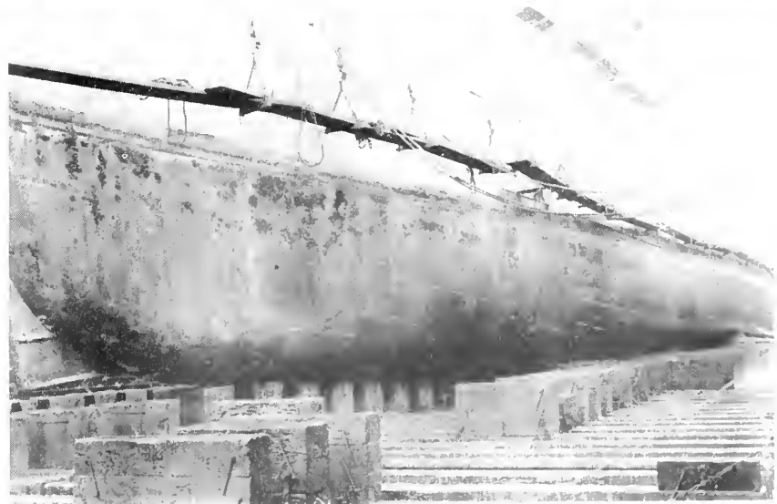
Fig. 1, top of page: Comparison cold plastic left, Old 15RC center and hot plastic right. USS Arctic, eight months waterborne.
