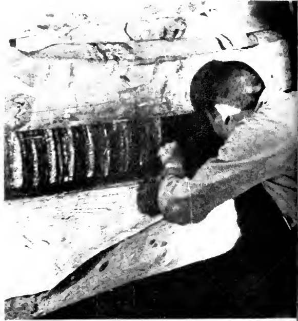
6 Old-fashioned method of pressing oil by a system of wedges. What is left is used for cattle feed.
