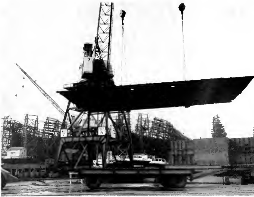
Like old times. (Well, not quite, but section lifts like this are not uncommon now that Oregon Ship is in production on the three luxury liners under construction for Alcoa.)
