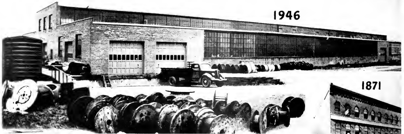
The Upson-Walton Company, Cleveland, manufactures wire rope, tackle blocks, boat fittings, accessories and brattice cloth in the modern plant. Inset shows original quarters of company in 1871.
