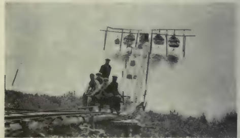
Crewe Bros. Fishery dock, showing the boats in their hoists with a loaded car being drawn up the bill by a natural gas engine in the fish house at the top.
