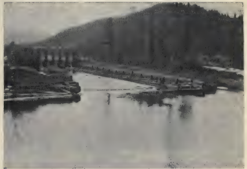
The Fish-way of Quesnel Dam, showing construction.
