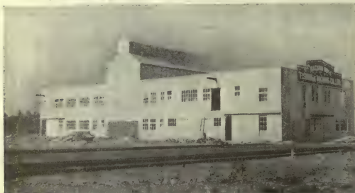
Watson, Bros. New Plant, Industrial Island, Vancouver, B.C.
