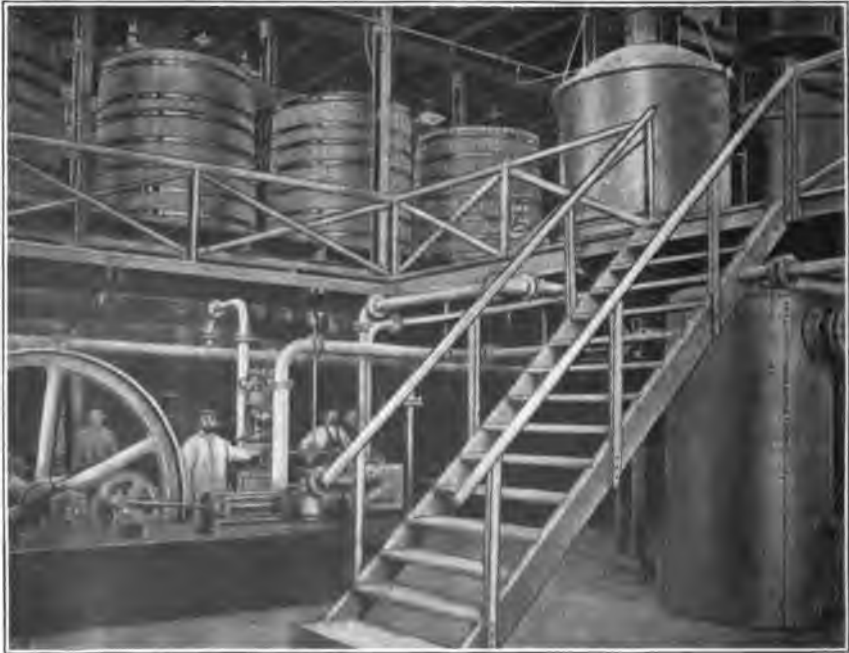
INTERIOR OF A QUEBRACHO EXTRACT FACTORY.
