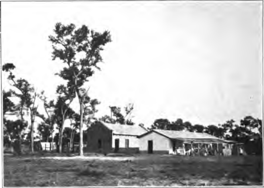
MANAGER'S HOUSE ON A QUEBRACHO ESTATE IN ARGENTINA.
