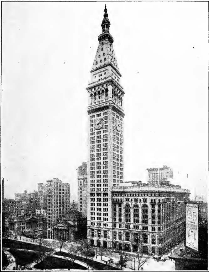
FIG. 120. The Metropolitan Life Insurance Building, New York. The chime consists of four bells, weighing respectively seven thousand, three thousand, two thousand, and fifteen hundred pounds, and tuned to D flat, E flat, F flat, and G.
