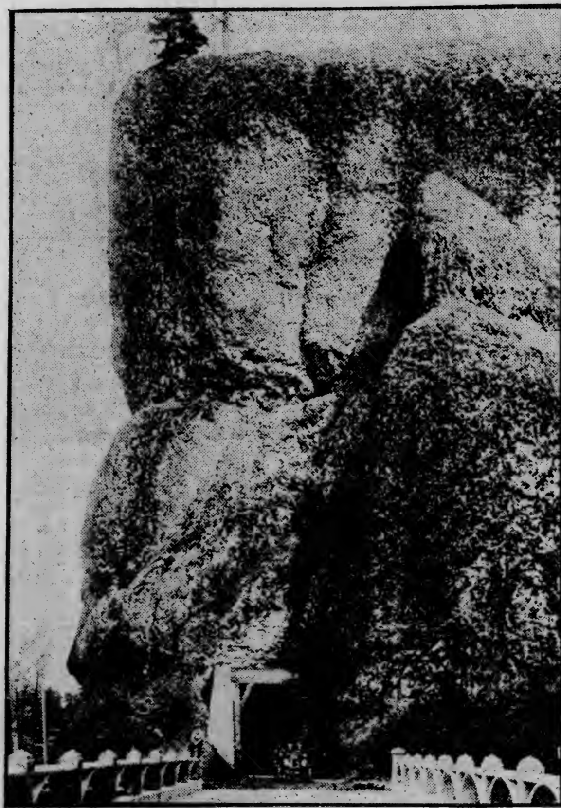
COLUMBIA RIVER HIGHWAY TUNNEL. On June 7 will be dedicated the new Columbia river highway, probably the finest automobile boulevard in the United States. This picture shows where the road was tunneled through a great rock barrier at Onocenta Gorge and carried beyond on a concrete bridge built over the river. The first forty miles of the road have cost $2,000,000.
