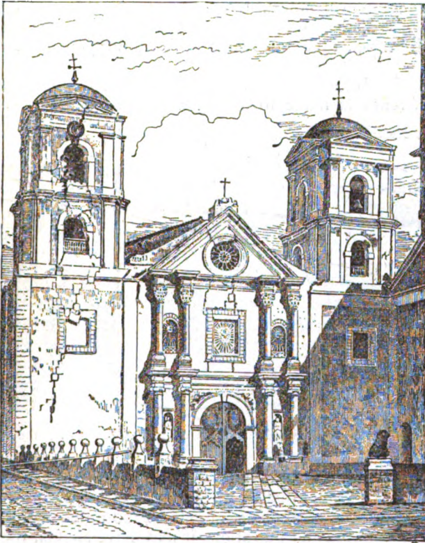
FIG. 3.—Church of St. Augustine, Manilla. Earthquakes of July 18–20, 1880.
